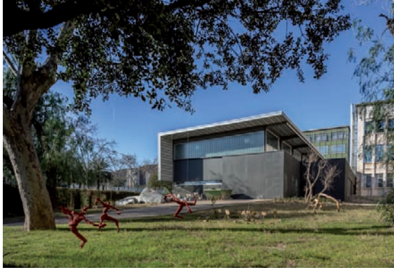
The new Faculty of Fine Arts building
