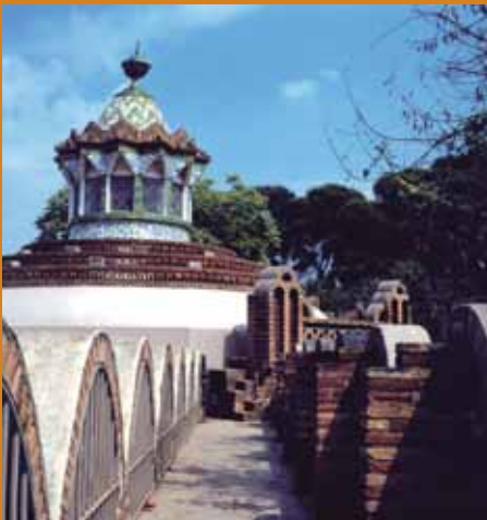
Arches and lantern seen from the roof of the stables
